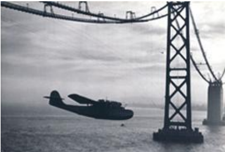
Pan American Airways Martin M-130 China Clipper flying under cables and guy wires of the San Francisco-Oakland Bay bridge on the inaugural flight November 22, 1935. Clyde H. Sunderland. SFO Museum. Gift of Thomas A. Northrop.
